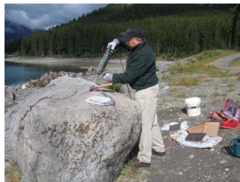
Archie Steacy drilling mounting holes in the granite boulder.
